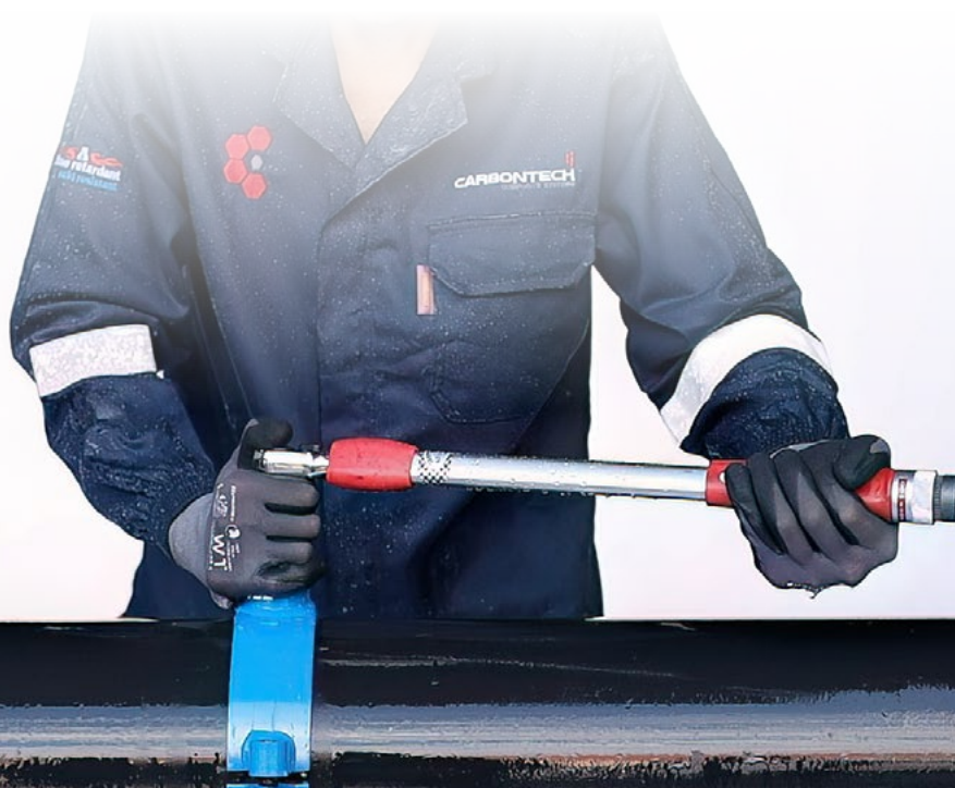
Viton Bung Shore A Hardness A60 Stainless steel backing plate
